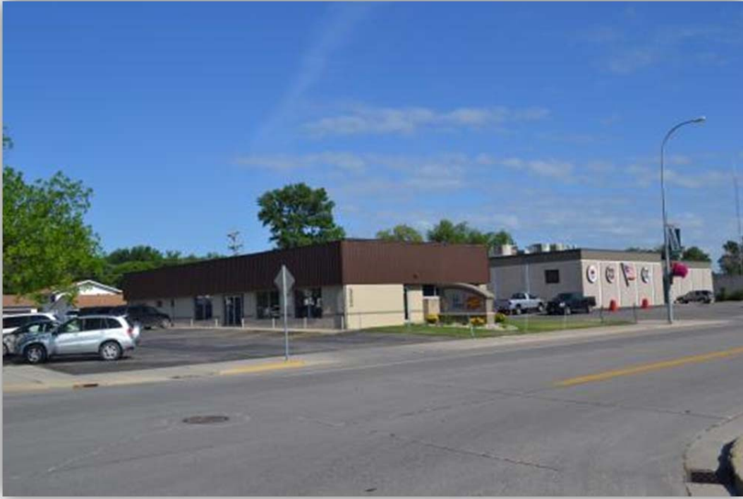
Facade Project Example: Off the Wall Advertising
