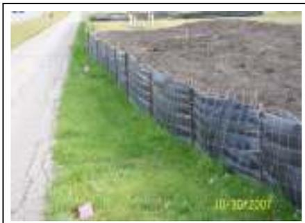
Silt fence with wire mesh backing
